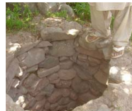
ABOVE Stones used in lining the soak pit. Photo: Syed Shah Nasir Khisro, IRSP, Mardan, NWFP, Pakistan.
